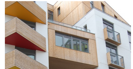
'Sustainable living' from choice of construction material to composting feature in Bioregional Quintain's 'One Brighton', UK. Big Hanna is listed in 'One Planet products'.
